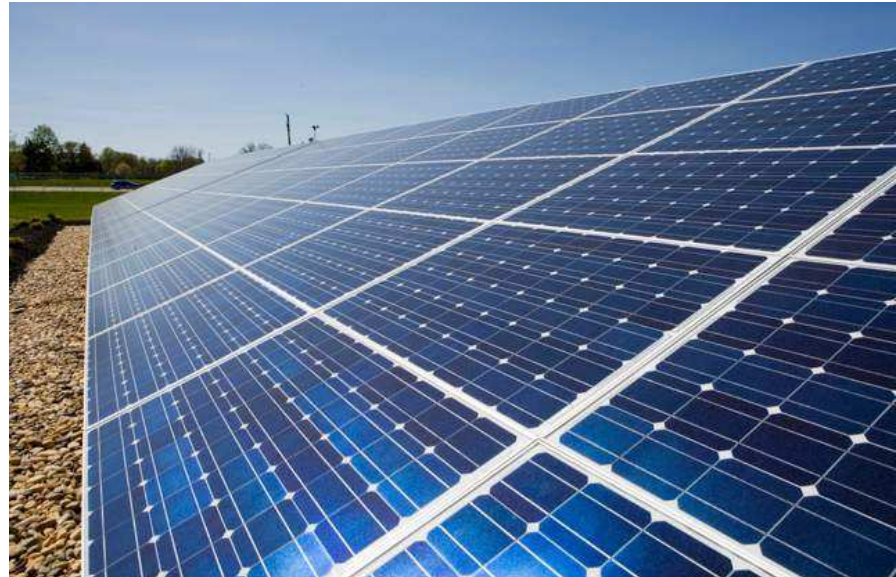
Proposal is to use standard Photovoltaic silicon cells.
